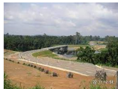
Road construction in Gabon
